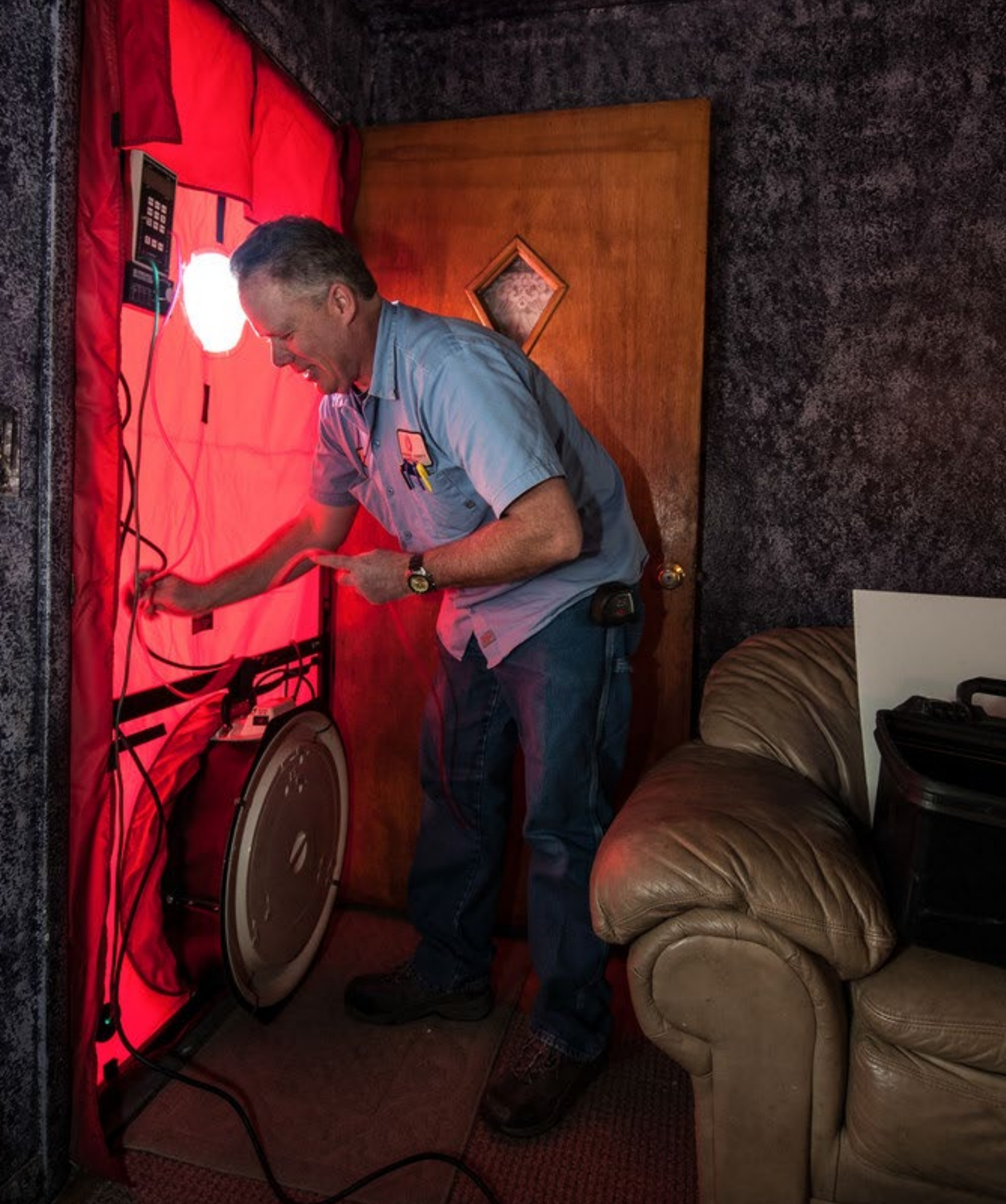
Ray Bowman, right, a Home Energy Professionals (HEP) Certifications Energy Auditor with Arapahoe County's Weatherization Division, performs a Blower Door Test, during an audit of a Thornton, Colorado home. (Photo by Dennis Schroeder / NREL)
